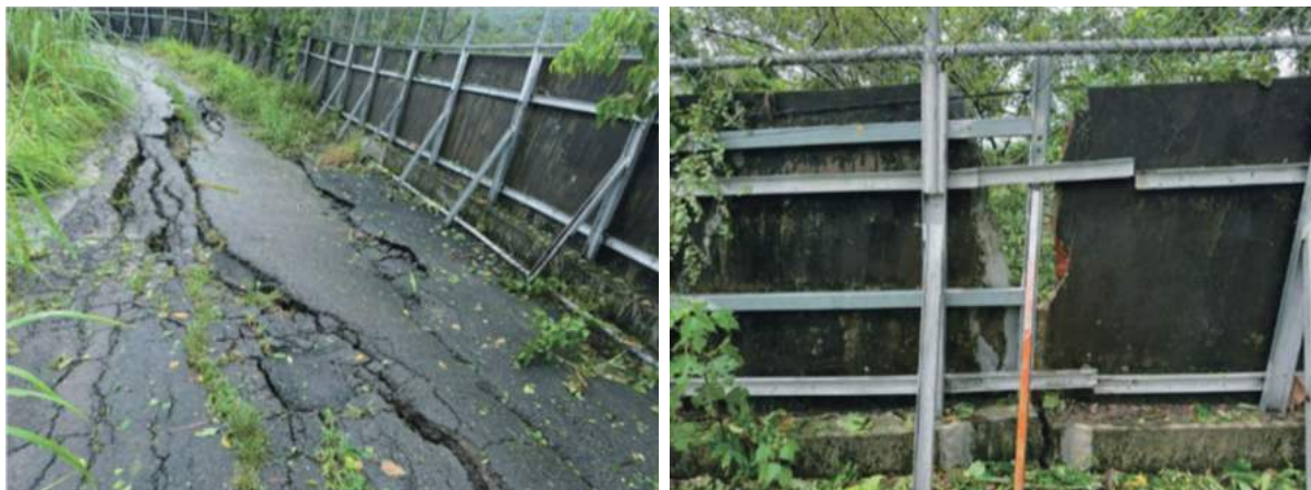
Figure 76 Collapsed Access Road and Damaged Retaining Wall Nansi Sanitary Landfill, Tainan City
